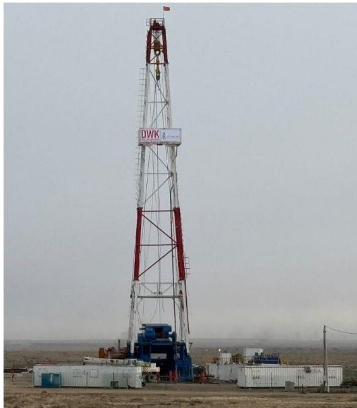
Figure 1: DWK rig in place for Jade's lateral well program
