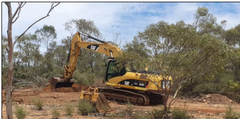
Figure 1: Excavator onsite beginning the trenching program.
