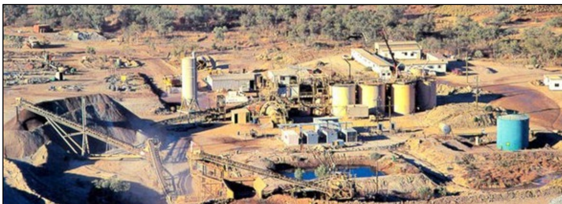
Figure 9 - Butchers Creek gold processing plant. Circa 1996.
