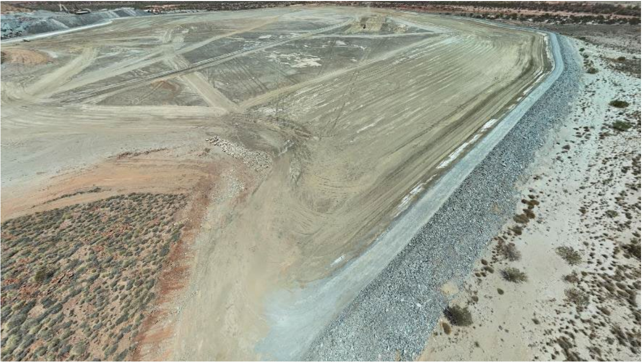
Figure 6: Showing the completed lift on the tailings storage facility facing East.
