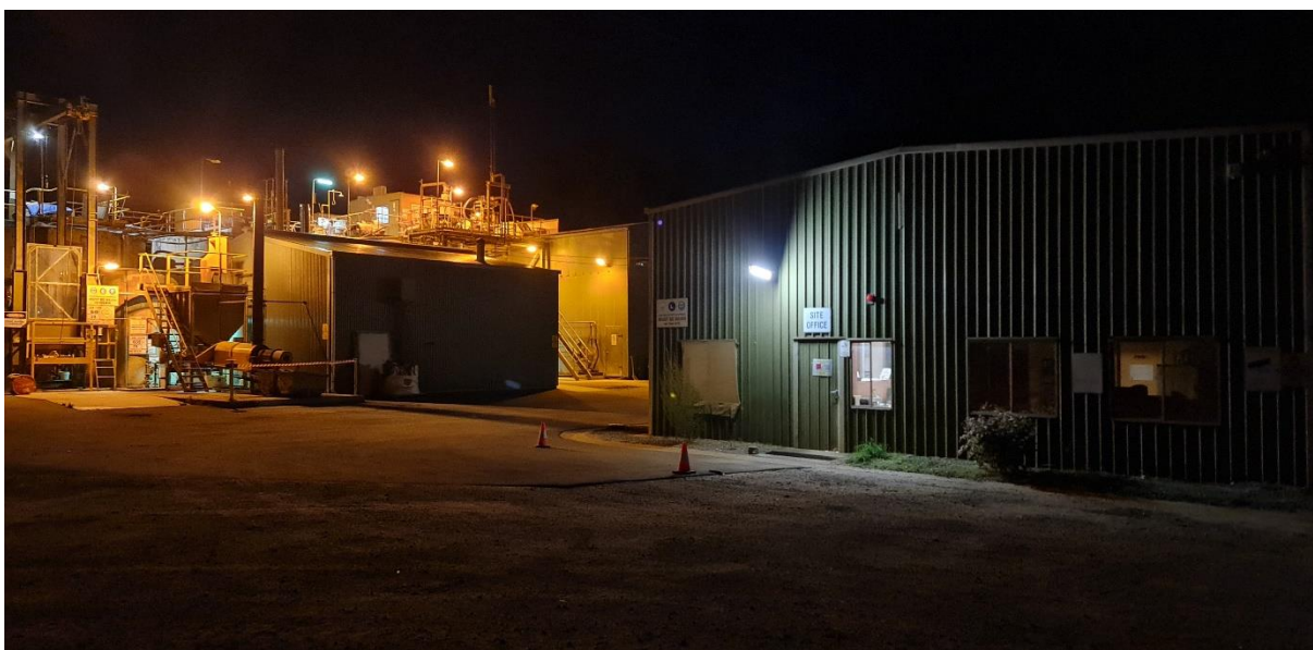
Figure 1: Maldon Gold Processing plant (front)
