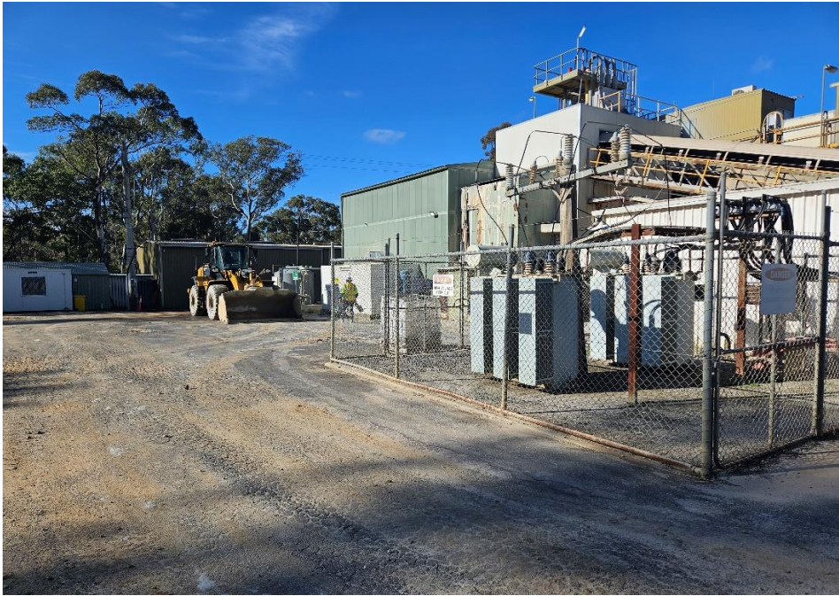
Figure 2: Maldon Gold Processing plant (rear)
