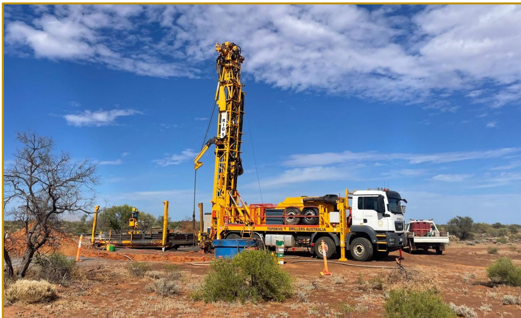
Figure 2. Core drilling at the Byro REE Project
