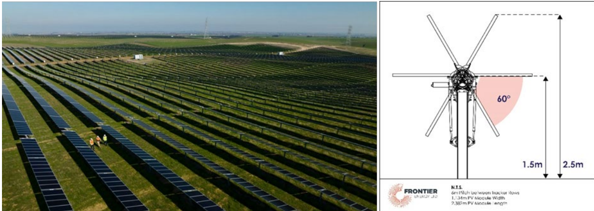
Figure 10: Typical solar farm arrangement with tracker
