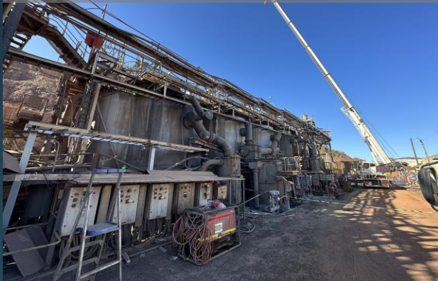
Repurpose of process plant as interim water treatment plant
