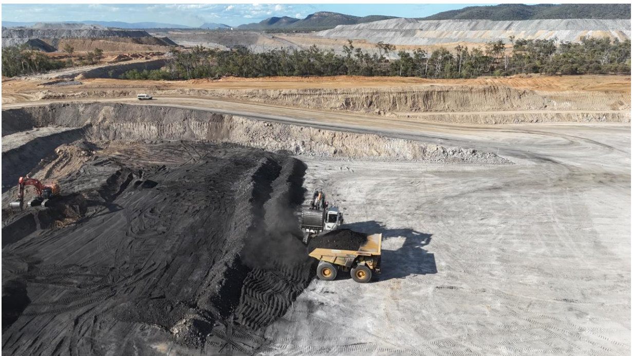
Figure 1: First run-of-mine coal being mined at Plumtree North
