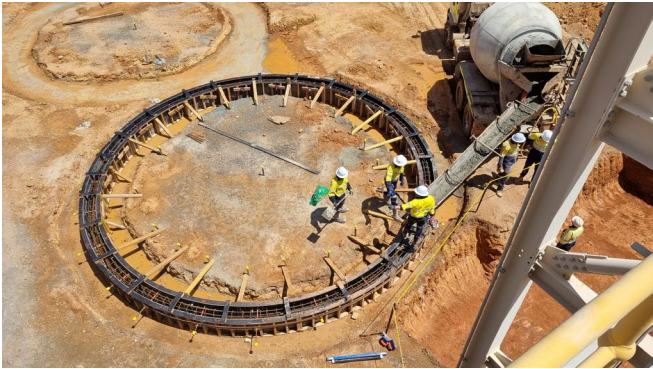
Figure 4: Concrete pour for tank ring beams, November 2024.
