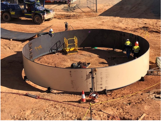
Figure 6: Fabricating tank skins, November 2024.
