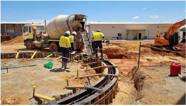
Figure 5: Concrete pour for tank ring beams, November 2024.
