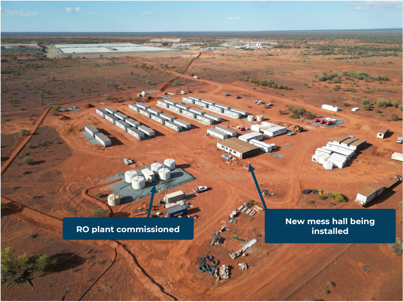
Figure 8: New installations at the accommodation village, November 2024.
