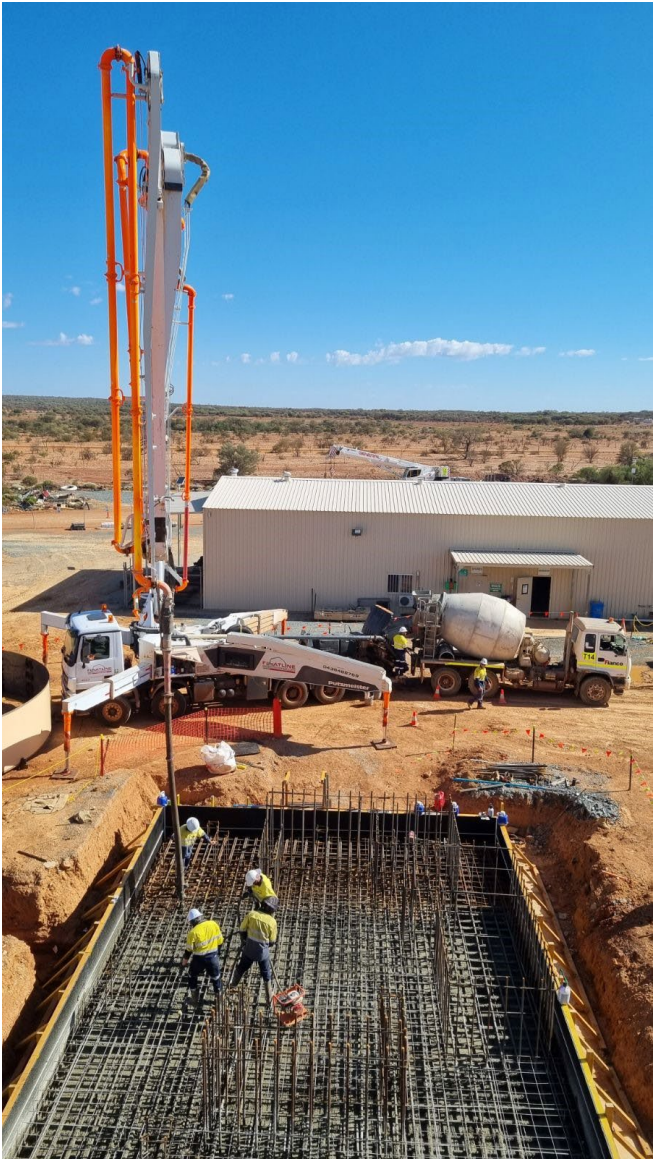
Figure 3: Concrete pour for ball mill foundation, November 2024.
