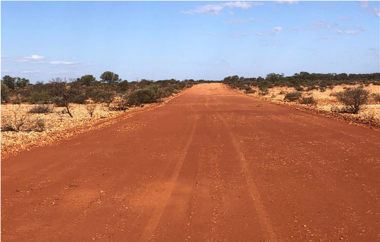
Figure 9: New 20km haul road, November 2024.
