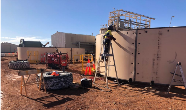
Figure 7: Fabricating tank skins, November 2024.
