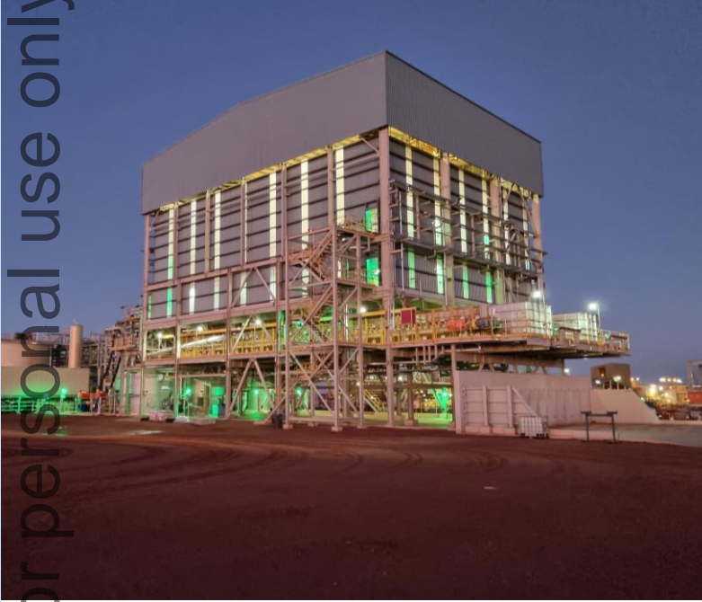
Mt Weld Expansion
