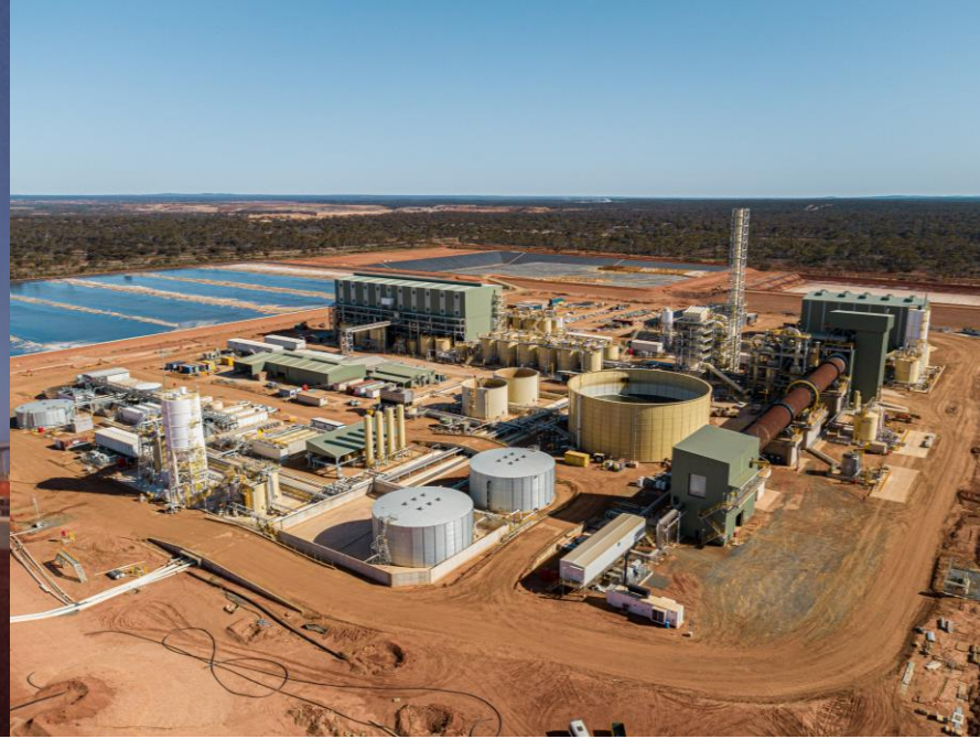
New Kalgoorlie Rare Earths Processing Facility
