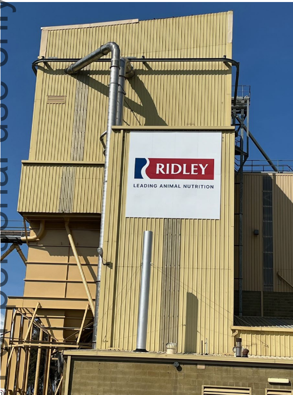
Carrick feed mill, TAS
