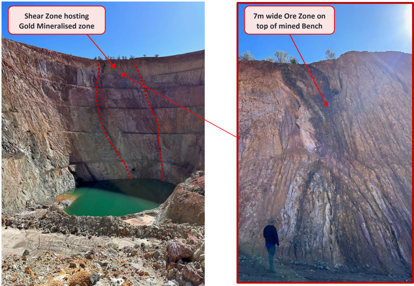
Figure 2 – Eureka Open Pit North Wall showing gold ore zone within shear zone
