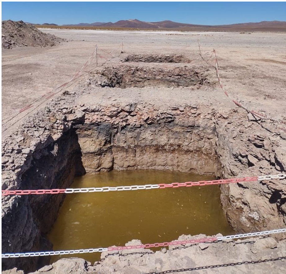
Figure 5. Sump wells have been excavated at JAM 24-05 well location on Cilon.
