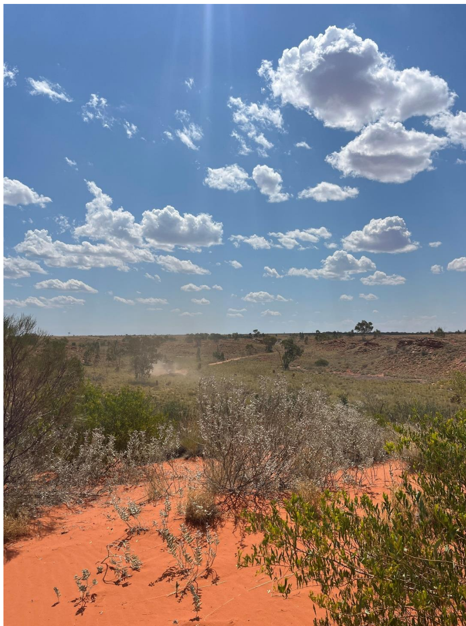
Figure 1. Access track being established at the Stansmore Project in West Arunta
