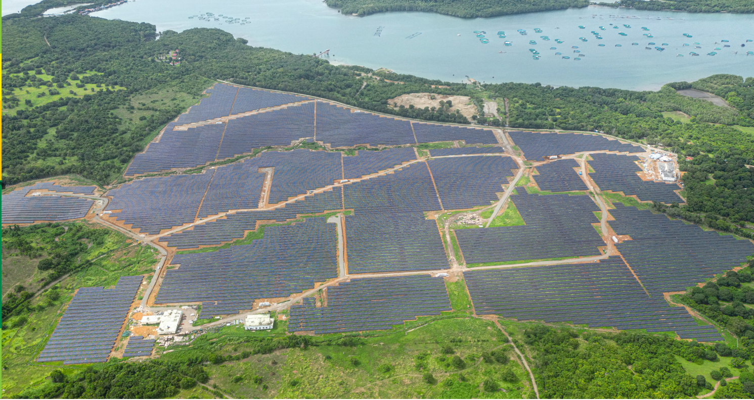
Gurin's 75MW solar power plant in Zambales Province, Philippines
