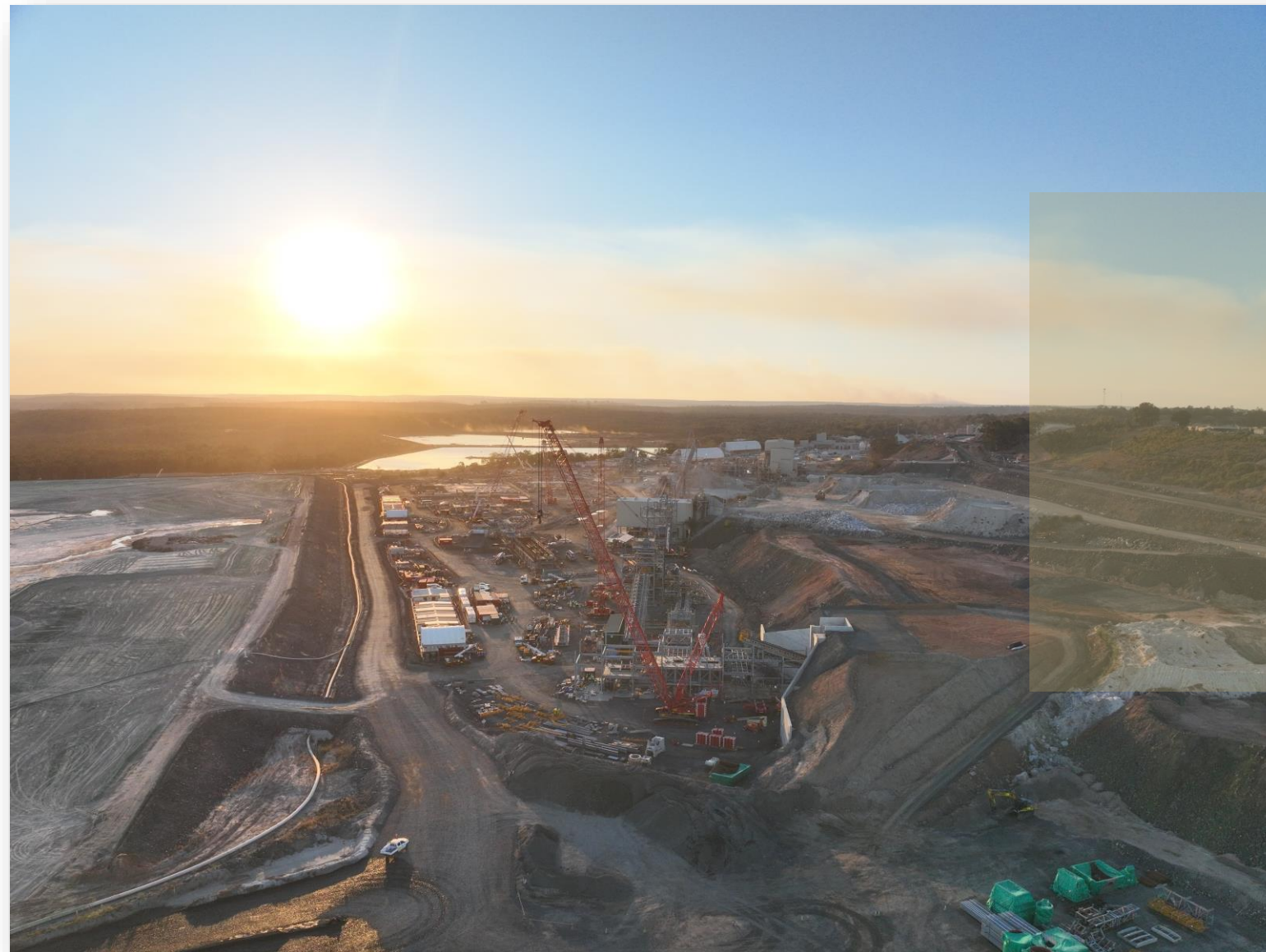
Chemical Grade Processing Plant #3 Project, Western Australia
