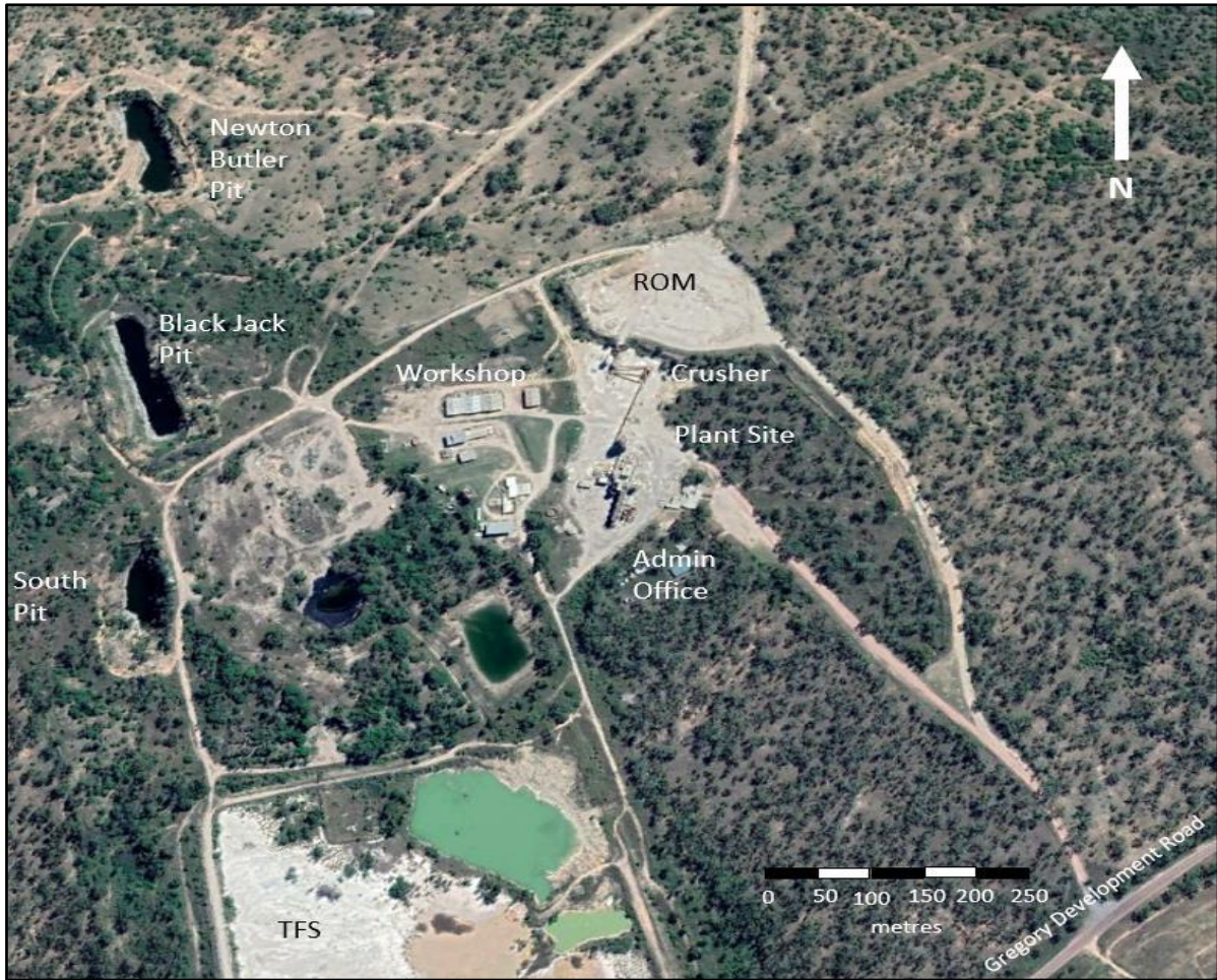
Figure 10: Black Jack site & surface workings
