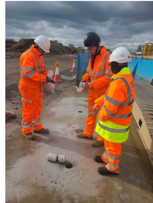
Slab coring and inspection of wear during Phase Two trials.
