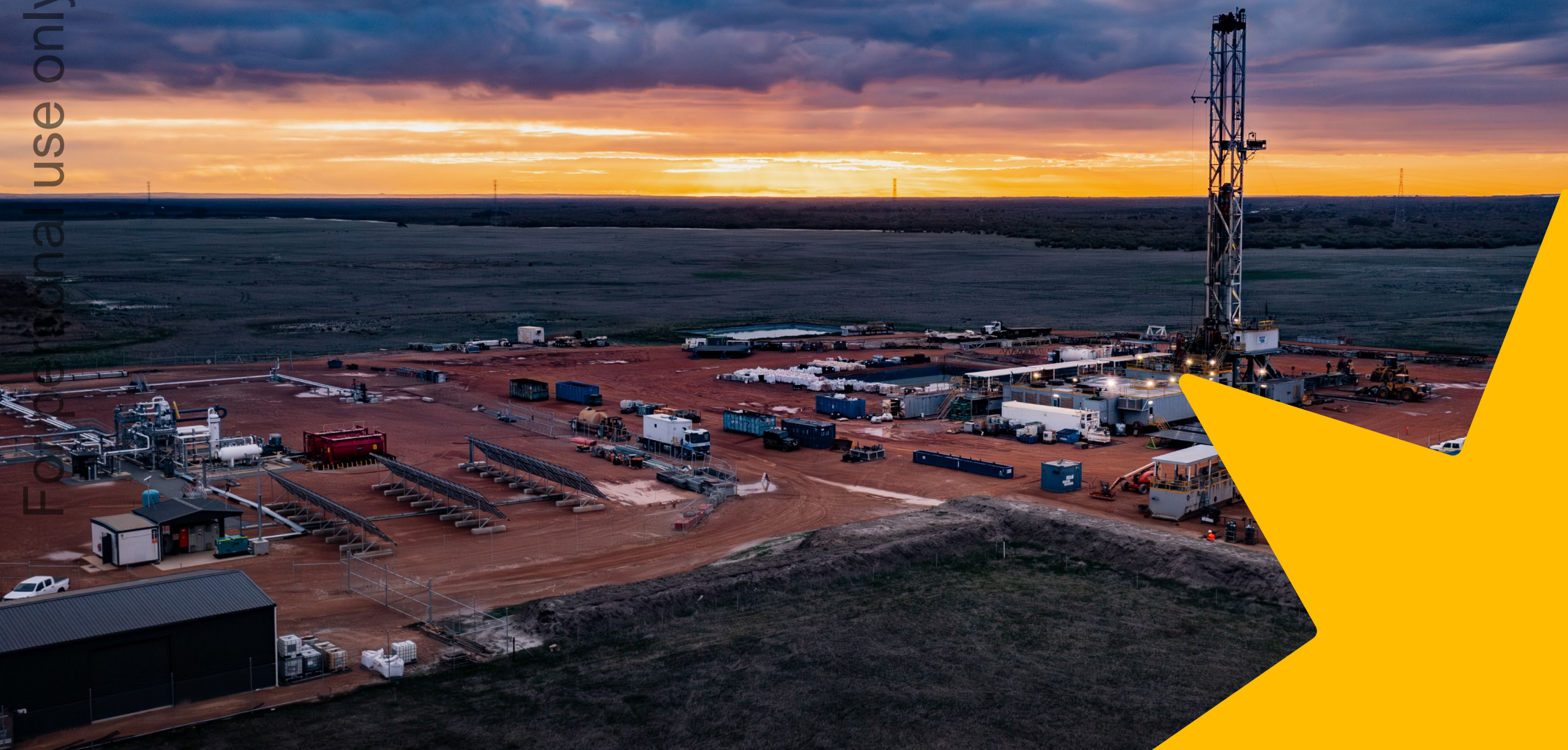
Walyering production operations and drilling at the W-7 discovery
