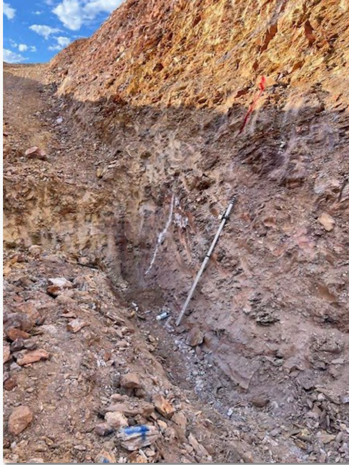
Picture 5. Current excavation progress in the ongoing bulk sampling program.
