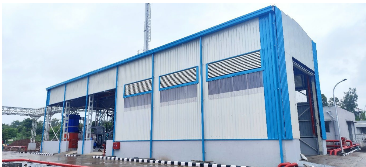
Figure 1 – part of the Panthera Graphite Technology (“PGT”) plant near Pune, India
