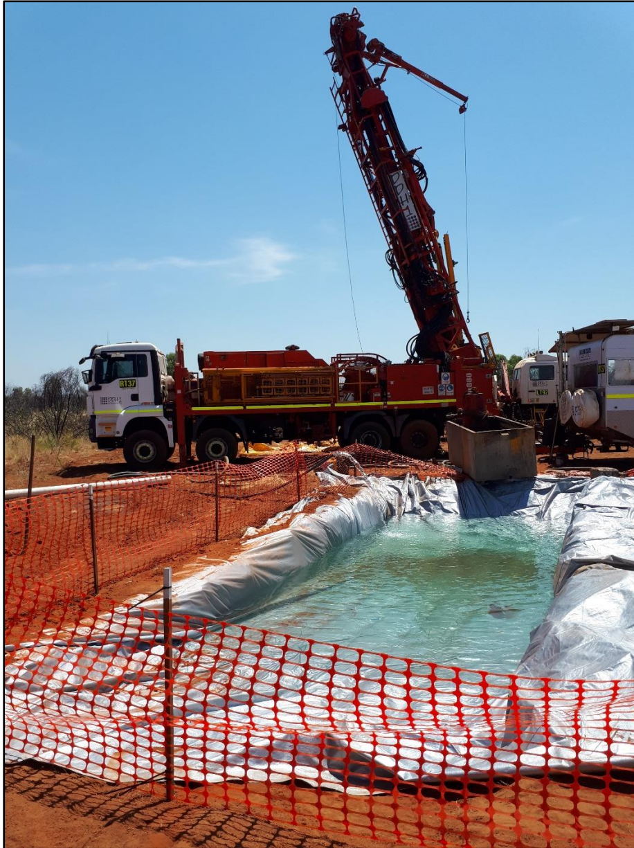
Figure 4. DDH1 drill rig set up at Leichhardt East.
