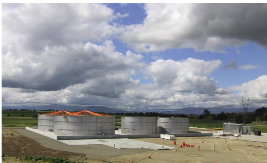
Image 1: YVW Bioenergy Project construction
