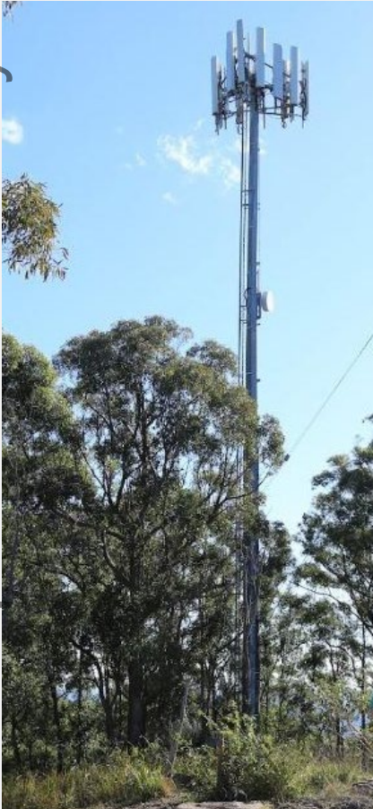
Securing mobile tower access
