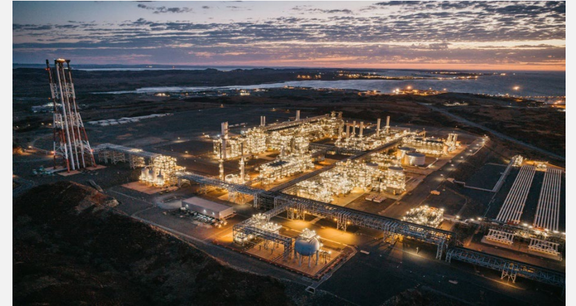
Major facility installed PIDS
