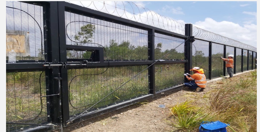
Security fence for rail corridor
