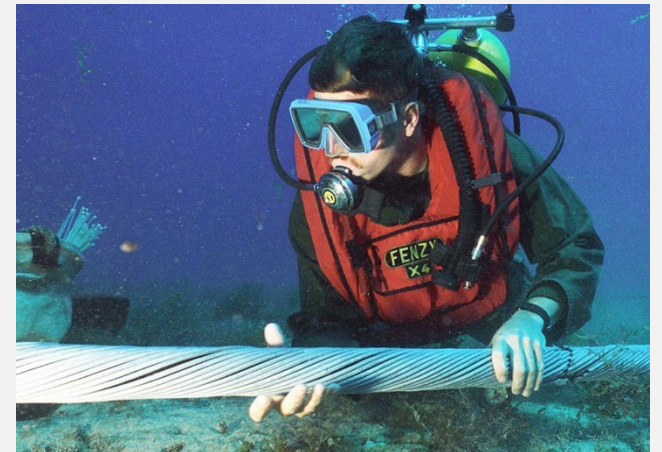
Monitoring of subsea telco cables
