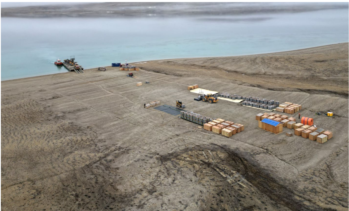
Figure 23: Photo of the Storm Project Marine Loading Area (MLA), on the coast of Aston Bay, Nunavut.
