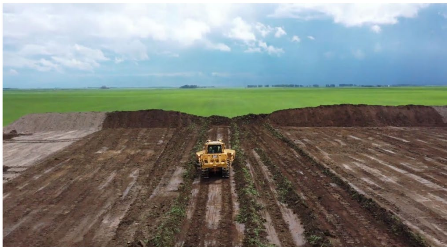
Figure 6: Construction of Pad #2
