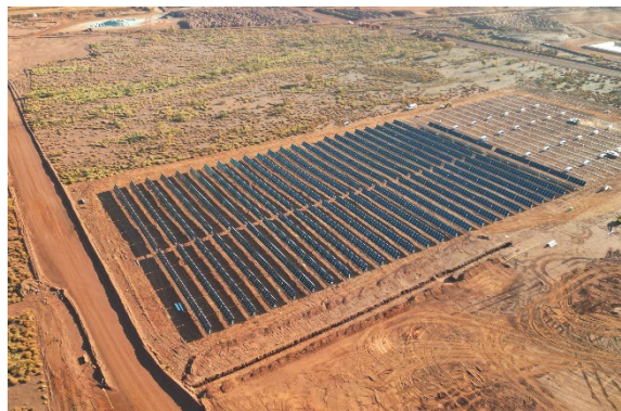
Solar array under construction at Ken's Bore
