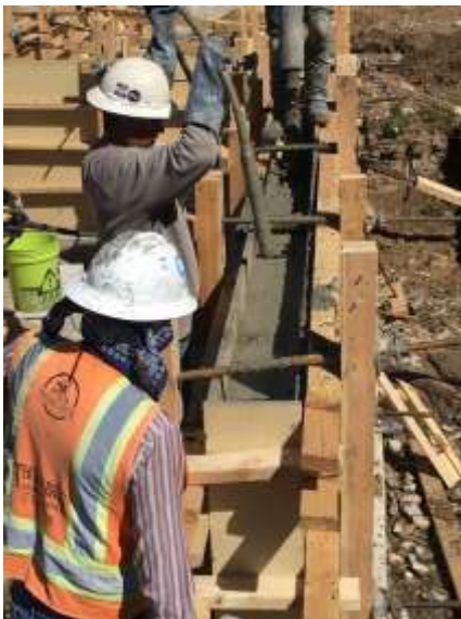
Figures 3 & 4 Second EdenCrete® Pz7 project- wall placement in Colorado
