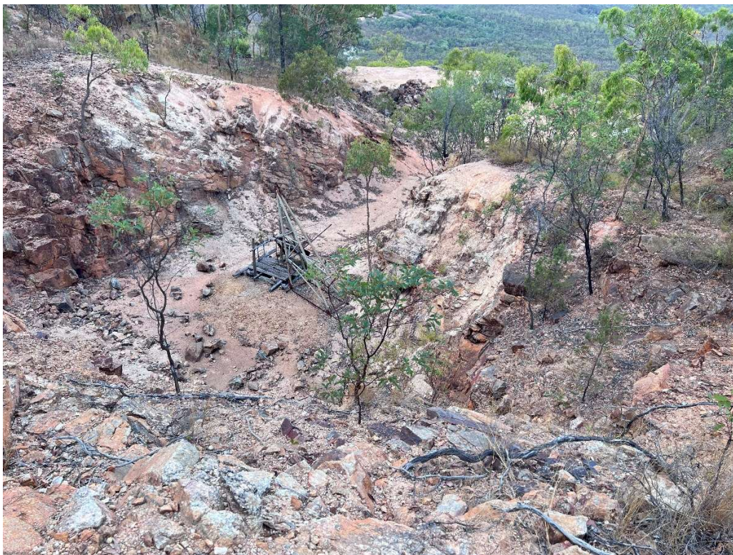
Figure 14. Photo of the historic Daisy Bell tin mine with shaft in foreground and open cut pit.
