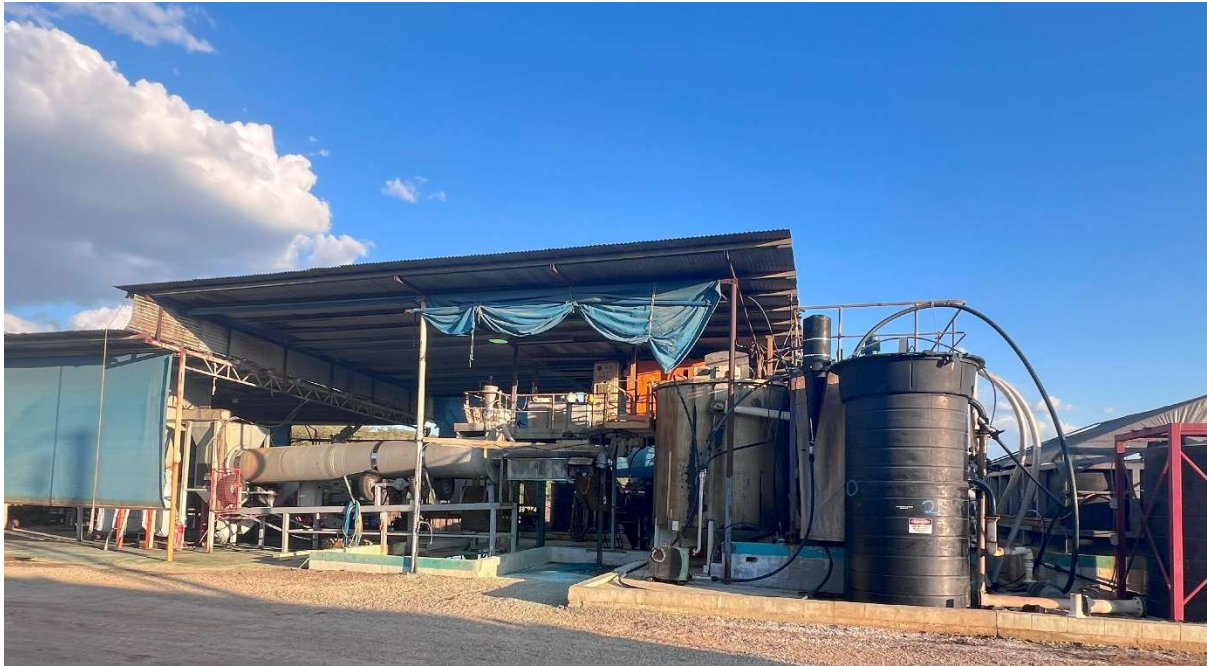
Figure 3. Photo of the copper sulphate pentahydrate production plant.
