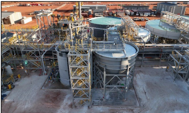
Figure 9: Water storage, thickening and concentrate settling
