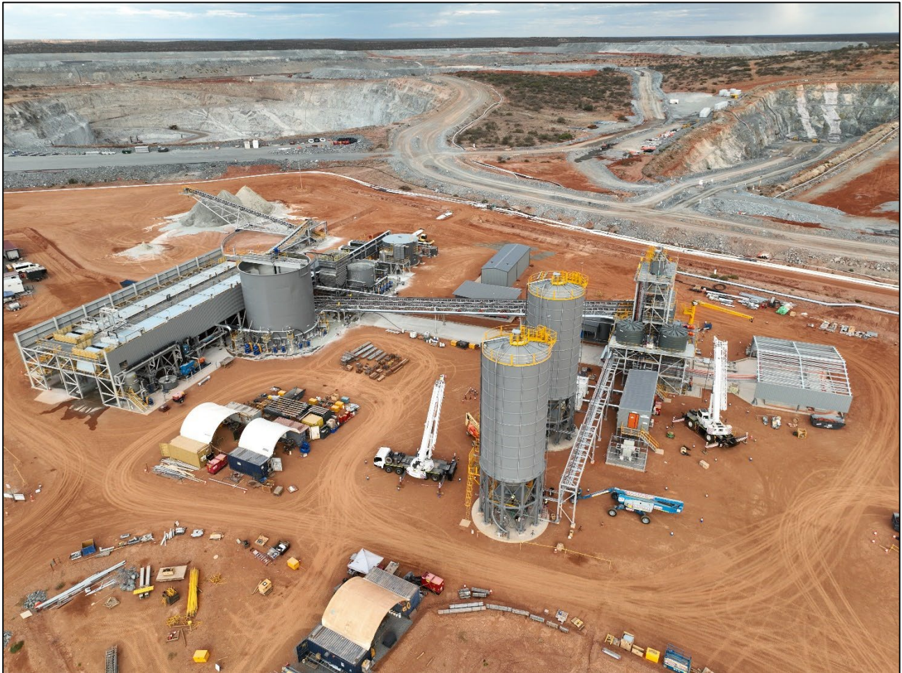
Figure 13: Aerial view of the paste plant
