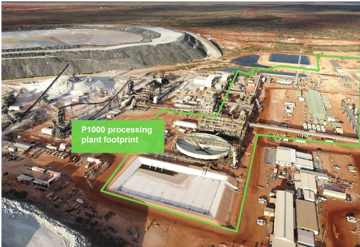
Figure 1: The P1000 Project as at 23 October 2024.
