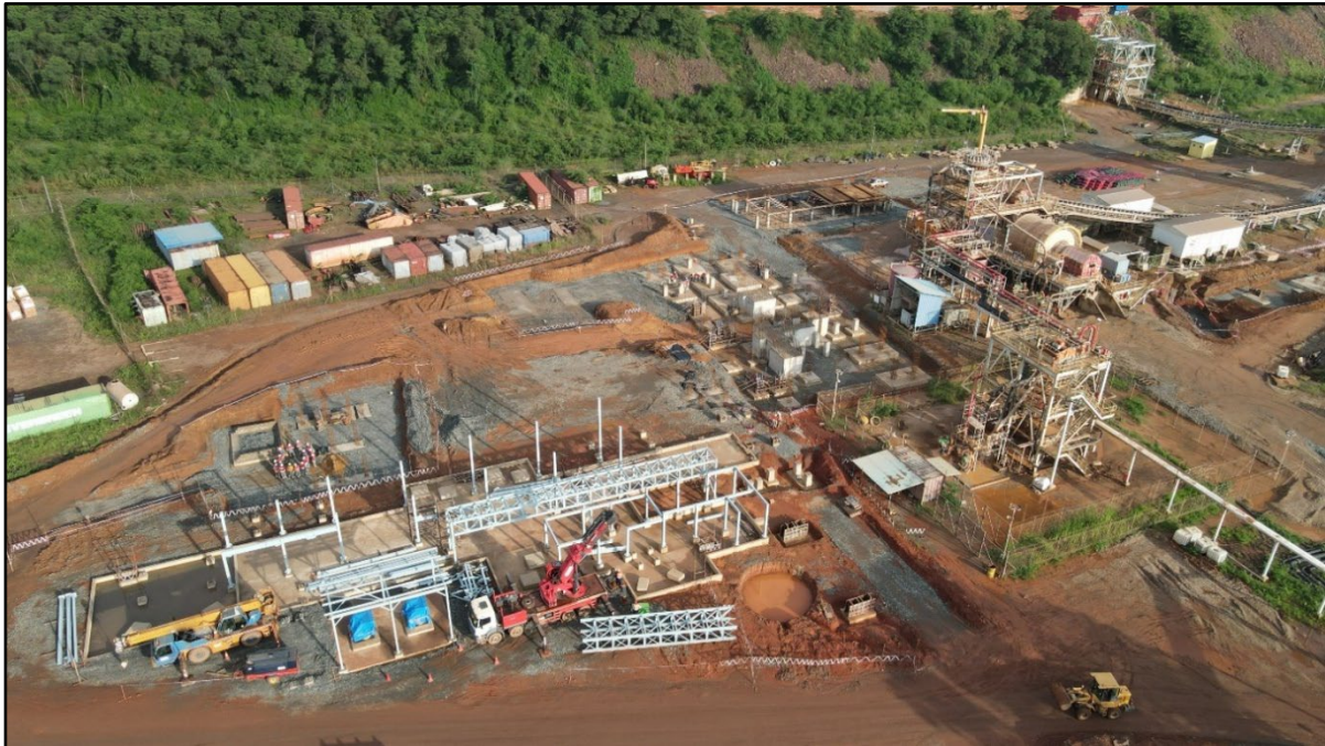
Figure 3: Ball mill and flotation area foundations
