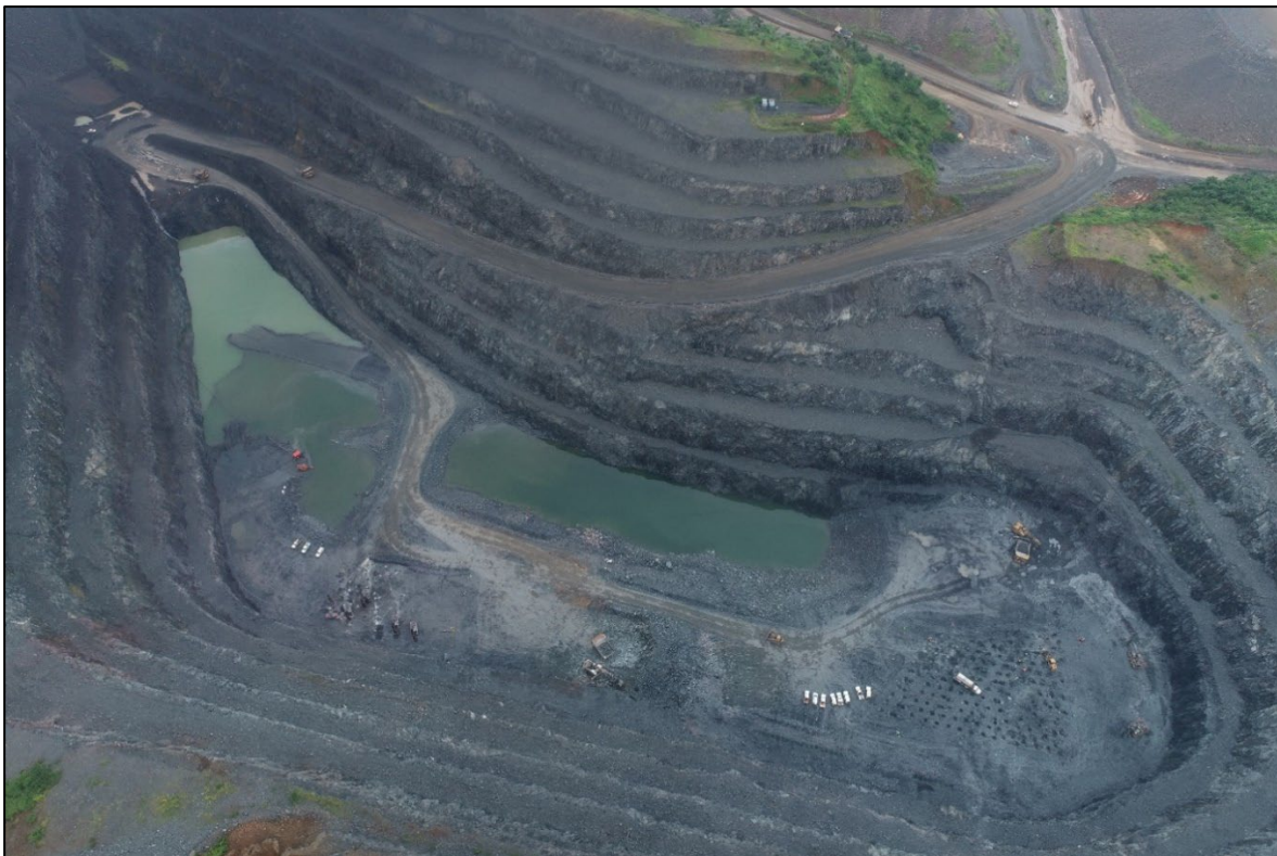
Figure 2: Inundation of lower areas where higher grades of the orebody are located
