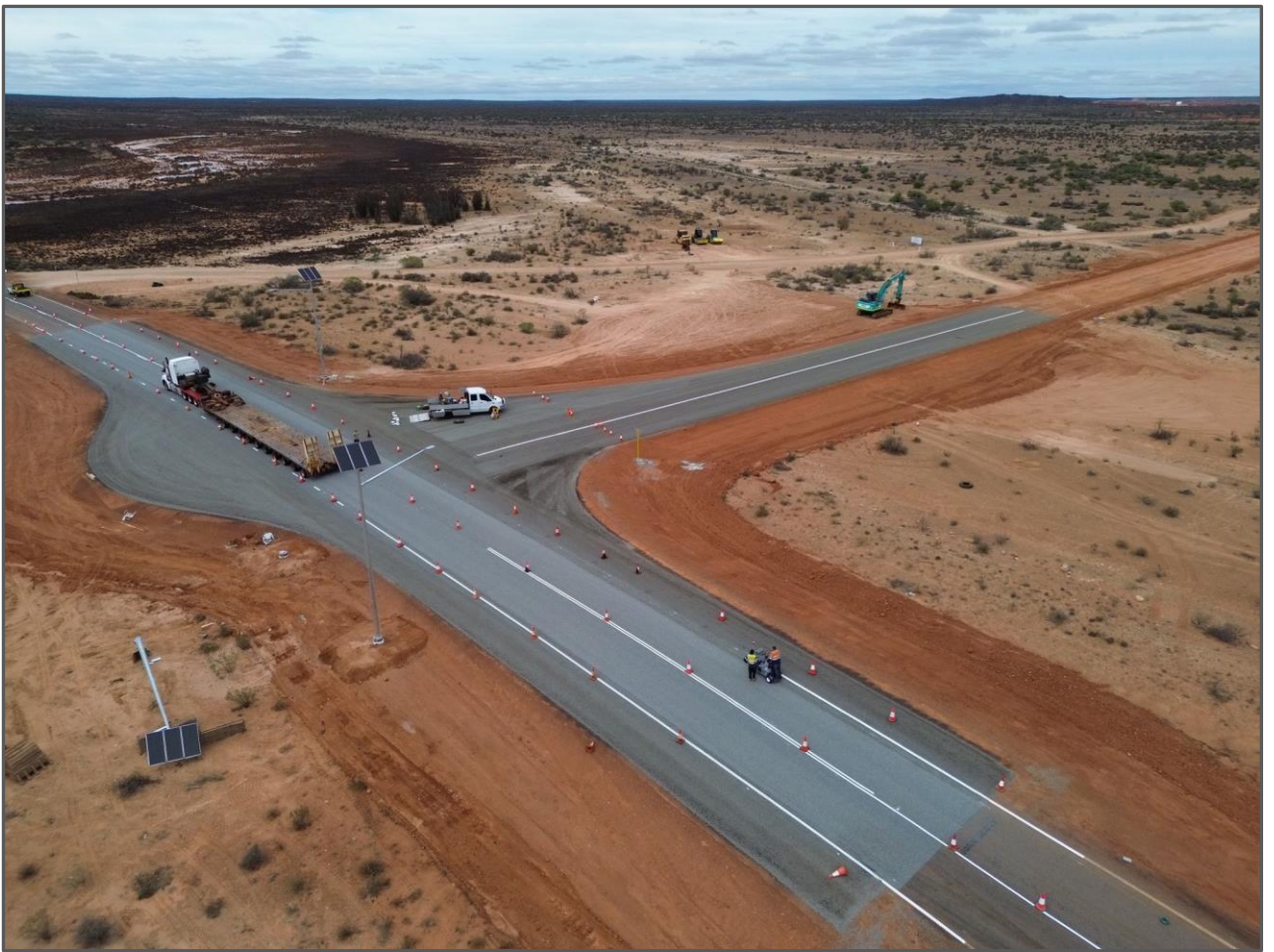
Figure 5: Cue Great Northern Highway intersection under construction
