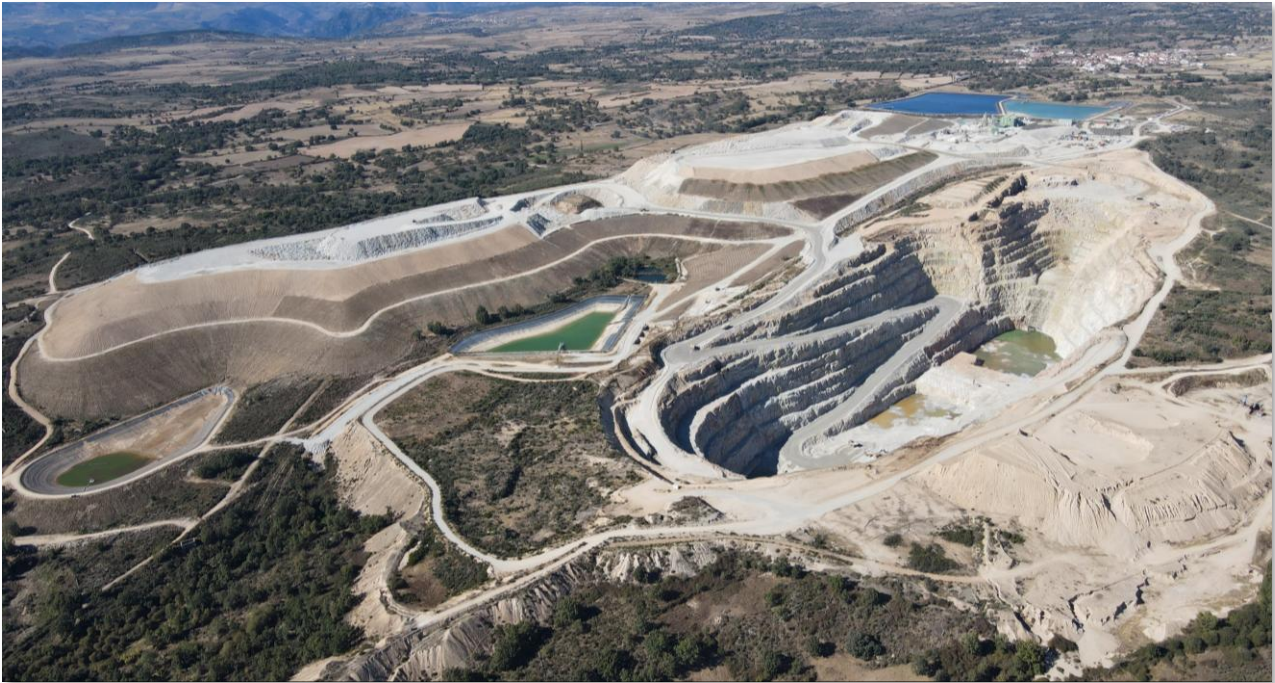
Pictured: The Barruecopardo Mine Open Pit (Spain) at the end of September 2024.
