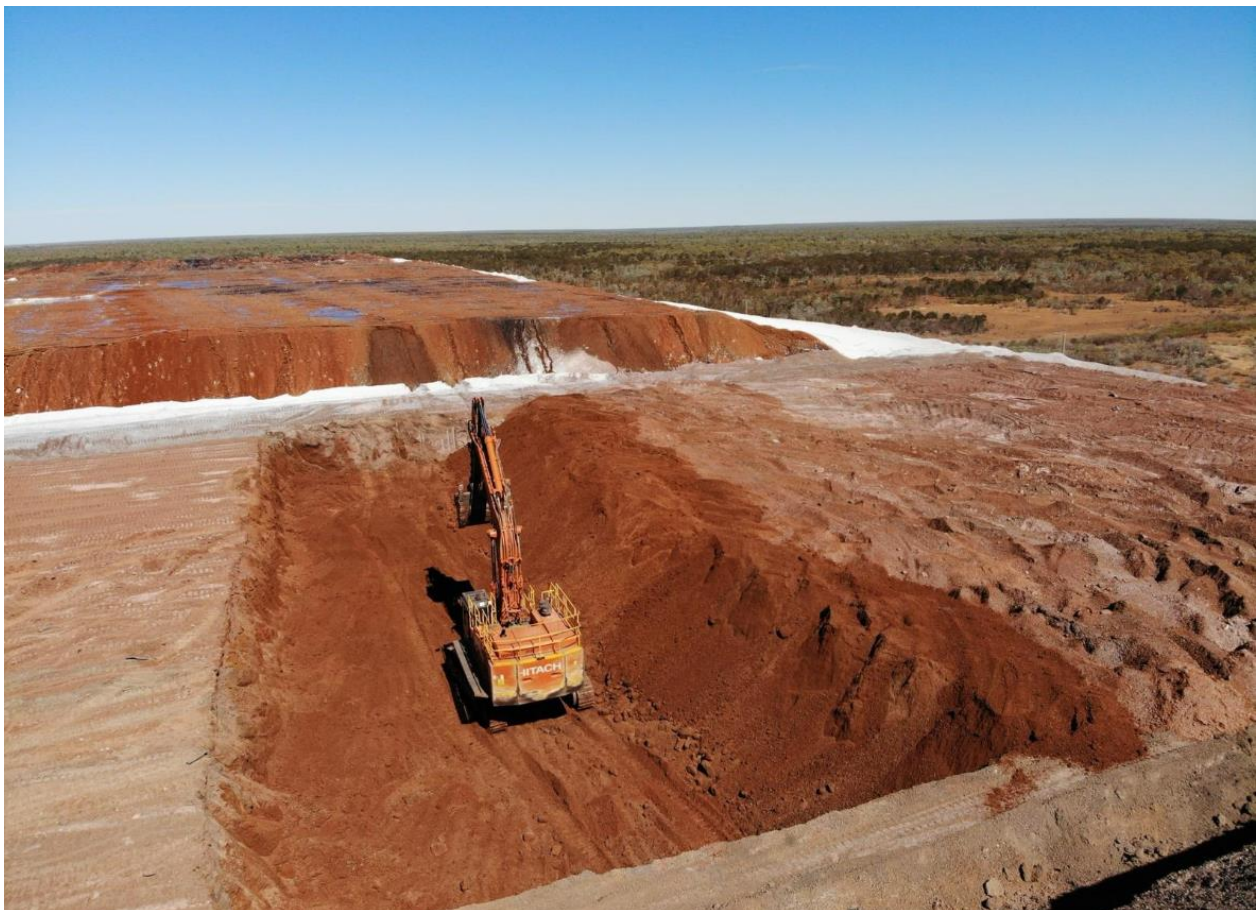
Photo 1. Excavator conducting remine operations in 2019
