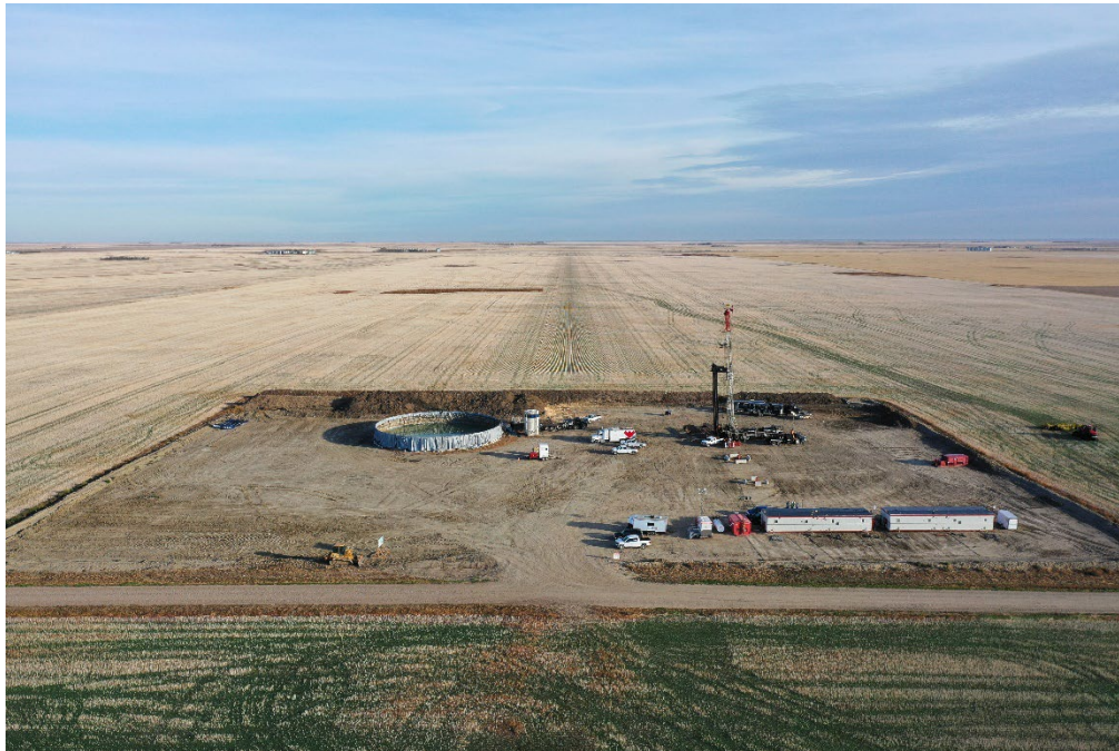
Figure 2: Service Rig at Pad #1
