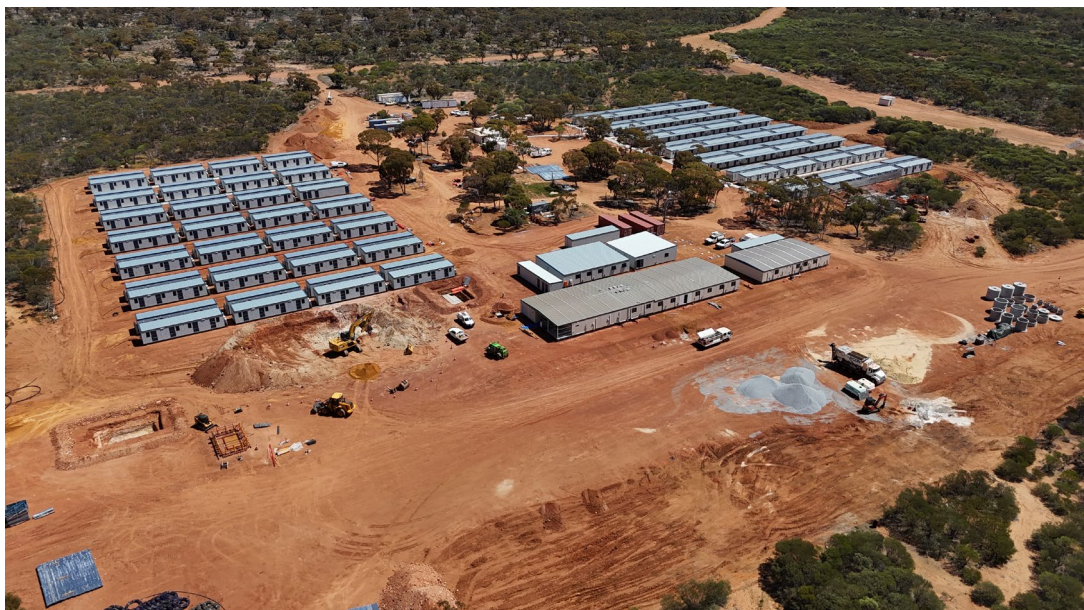
Mt Gibson Gold Project – accommodation village installation
