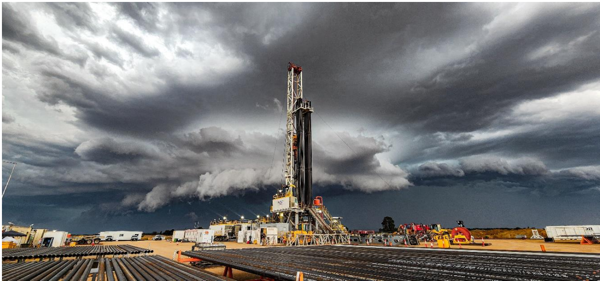
Image 1- Canyon-1H well site
