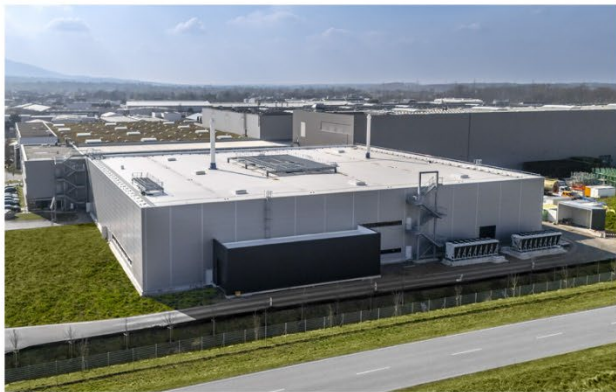
Figure 4 – Mercedes-Benz LiB Recycling Building, Kuppenheim Germany.
