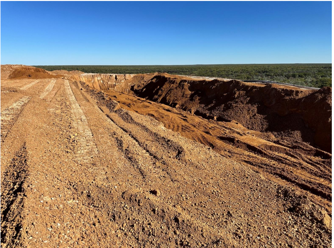
Figure 1. Pad 2/3 Re-Mine Operation at commencement.
