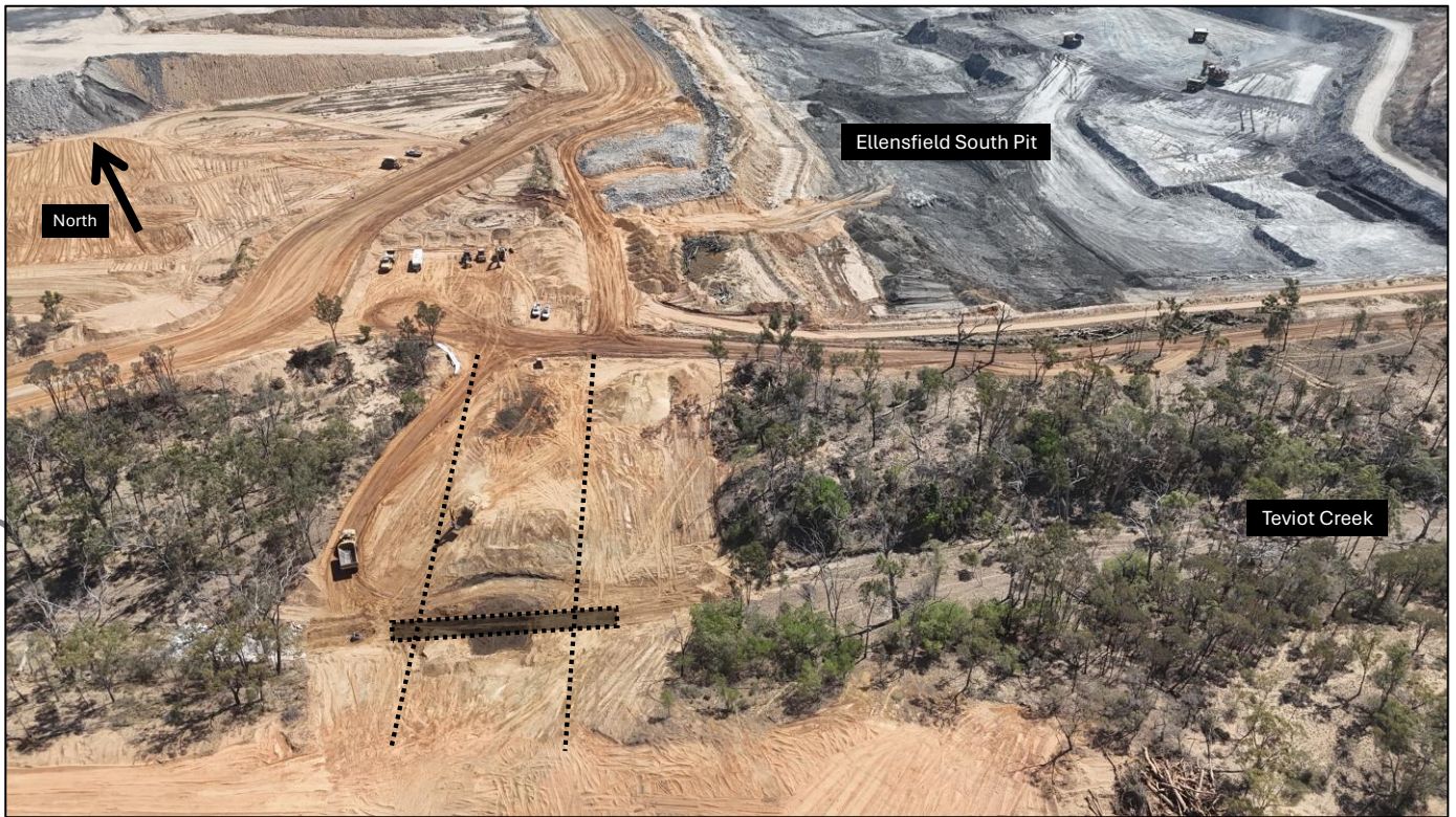
Figure 2: Teviot Creek Crossing Construction (looking north)
