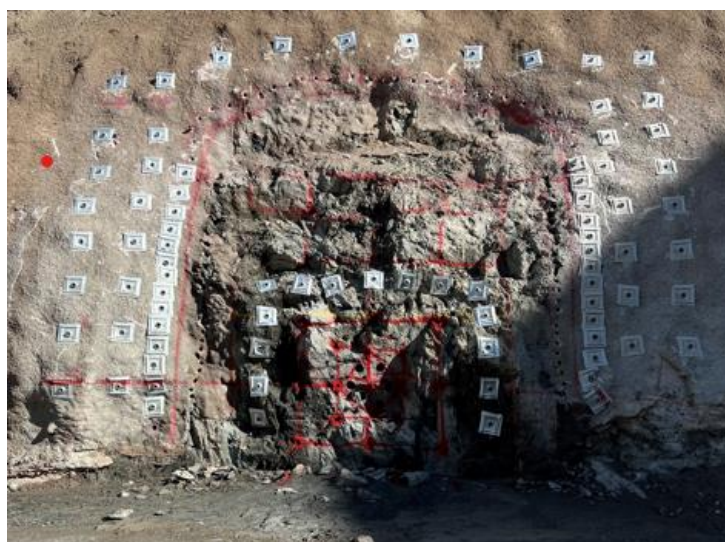
Figure 2: First cut of the Rosemont Stage 3 ventilation portal.
