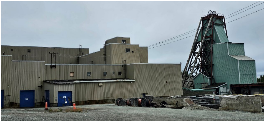
Figure 6: View of the Chibougamau processing facility and Copper Rand shaft.
