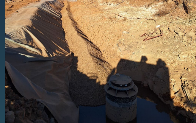
Interception sump (in progress)
