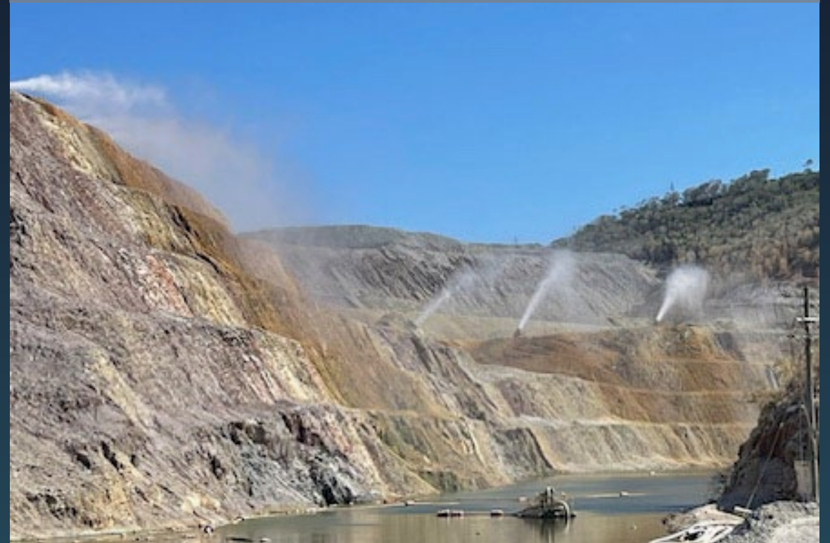
Mechanical evaporators at Esperanza Pit ('EPit')
