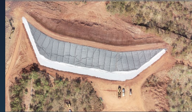
Enhanced water diversion infrastructure (complete)
