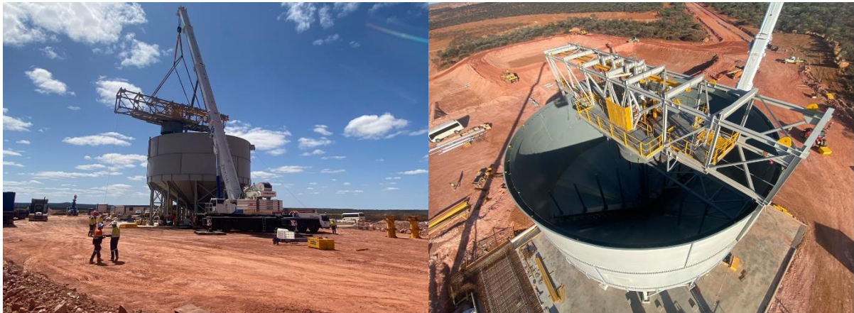
Figure 7: TSF 4 thickener assembly
