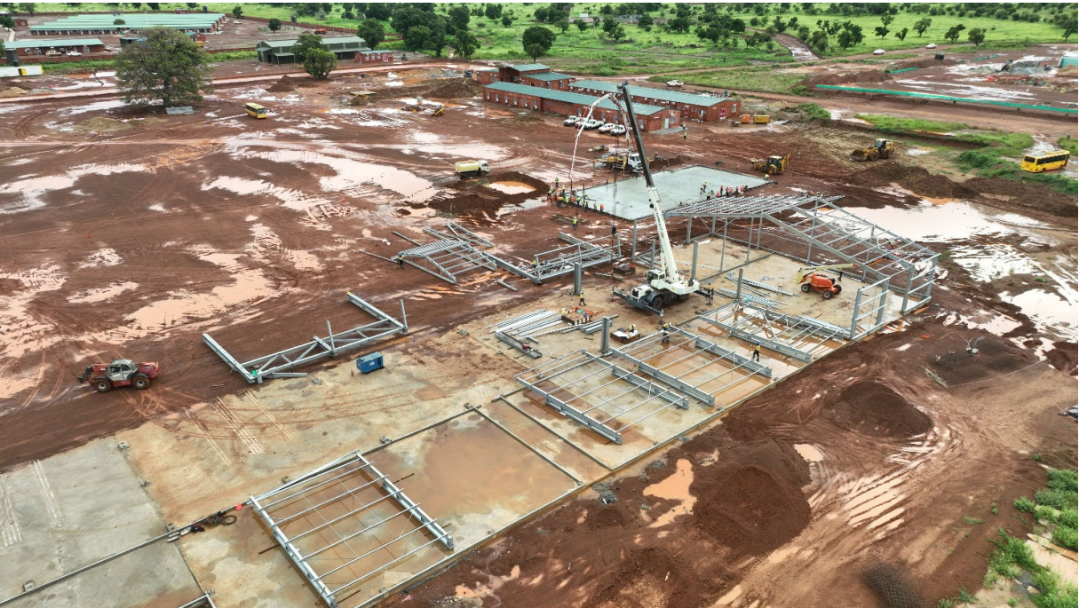
Kiaka Mine Services Area (HV Workshop & Offices)
