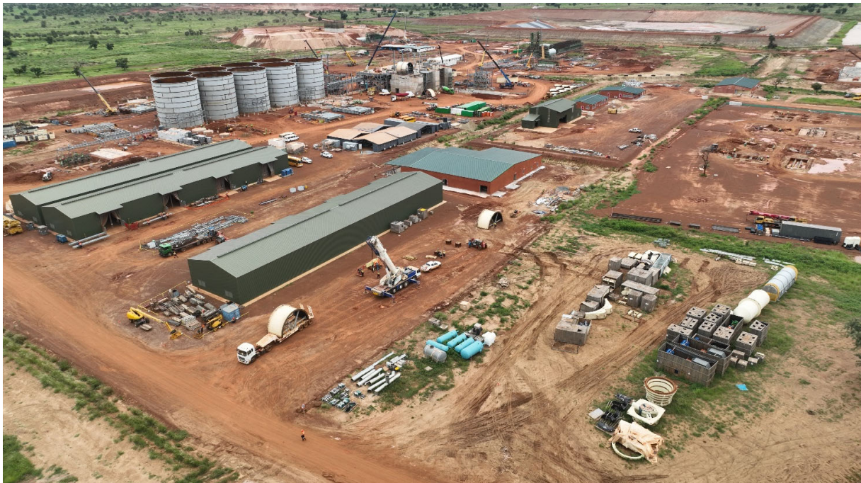
Kiaka Plant Overview
