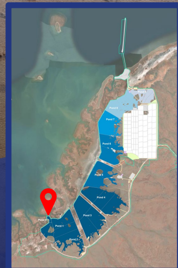
Seawater filling ponds 0 and 1
