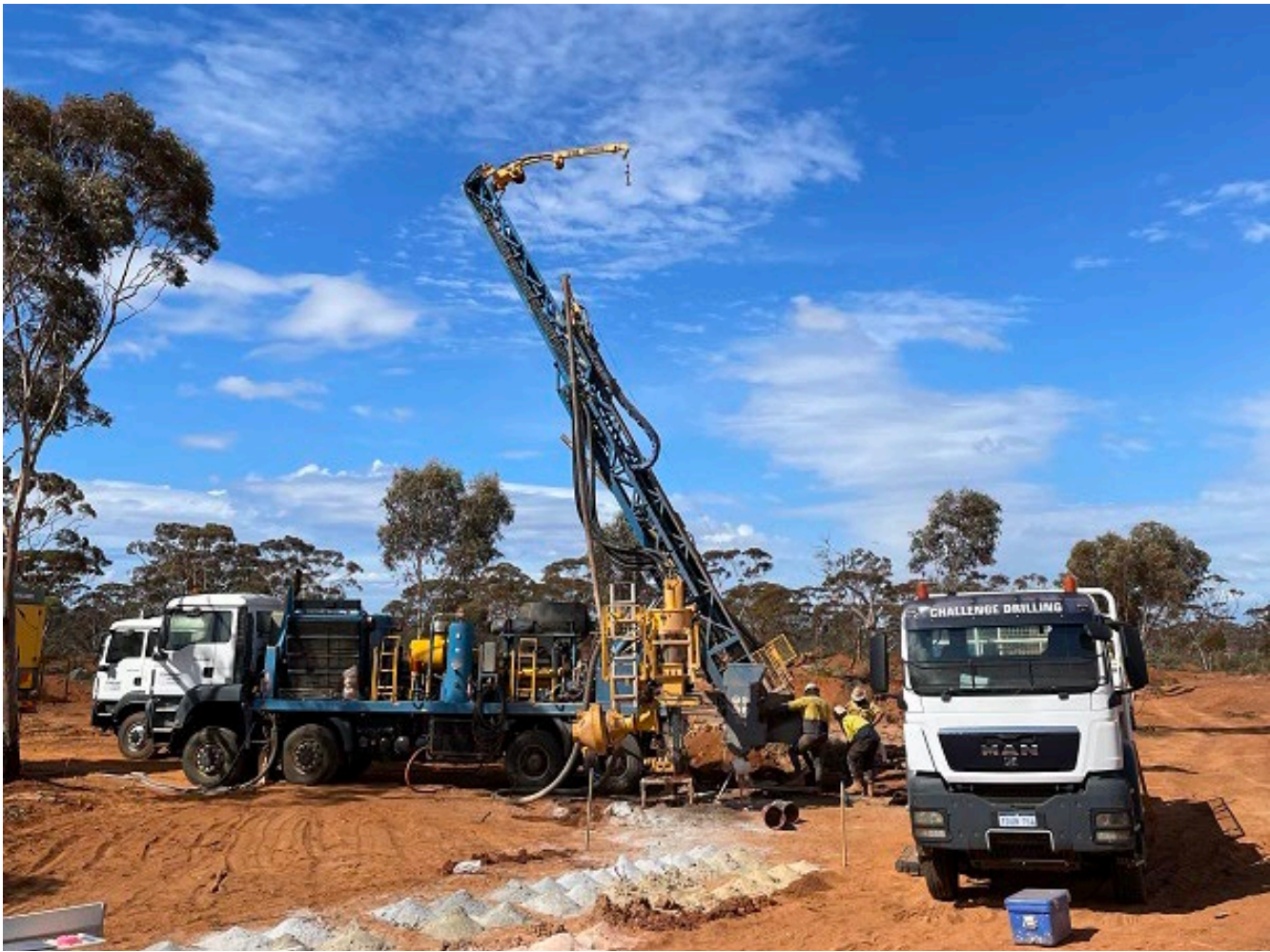
Image 1 – Theia In-Fill Drilling.
