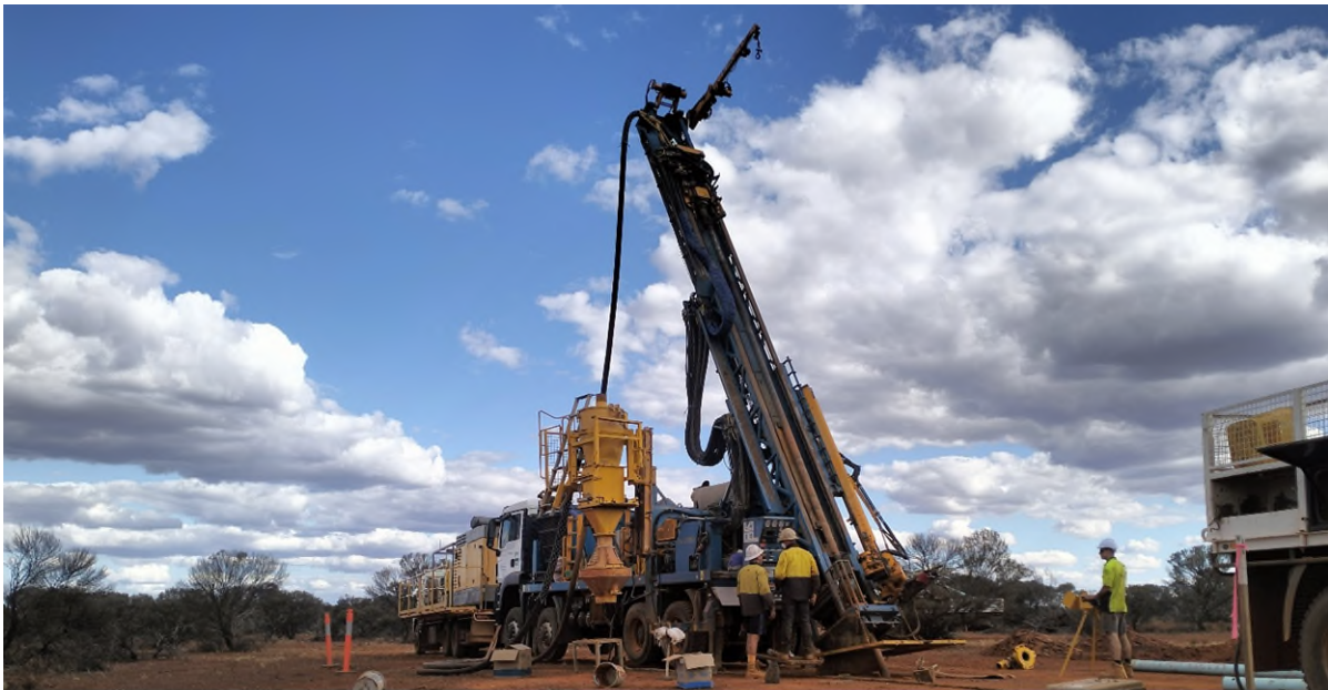
Figure 1, Challenge drilling onsite at Swiftsure with RC rig
